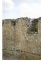
SaZwe.I, Burgmauer (Detail), DI008226, BSV-
