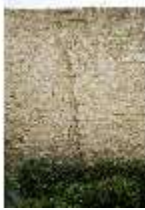
SaZwe.I, Wehrmauer (Detail), DI008225, BSV-
